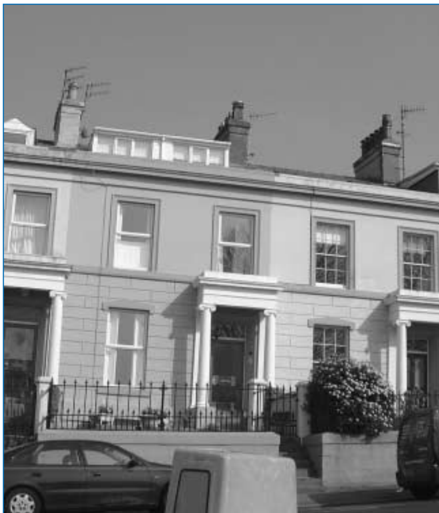
Housing in the Corkickle area of Whitehaven, has been refurbished through the Single Regeneration Budget (SRB)
